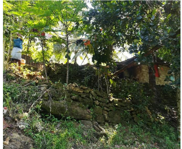
Figure 04 (b) – Houses locate at the potential slope failure location.
