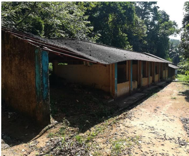
Figure 04 (c) – Abandoned School building due to landslide threat.
